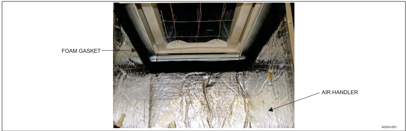
FIGURE 4: Gasket Location
